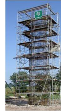
This upright for a railroad bridge is constructed of steel mesh and concrete.
