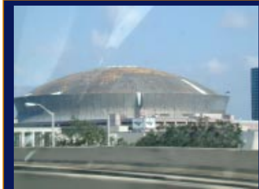
View of the superdome after hurricane Katrina.
